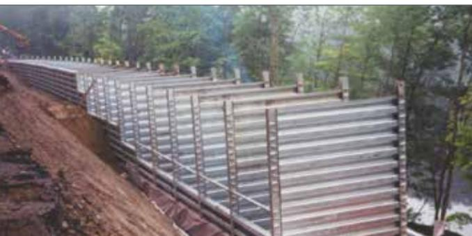
**Application:** Gravity-Type Retaining Walls for Mining Use
