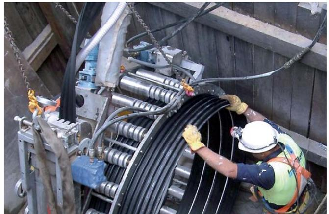
*SPR™ PE is a spiral wound, steel reinforced HDPE that is heat-fused to form a structural pipeline rehabilitation product.*
