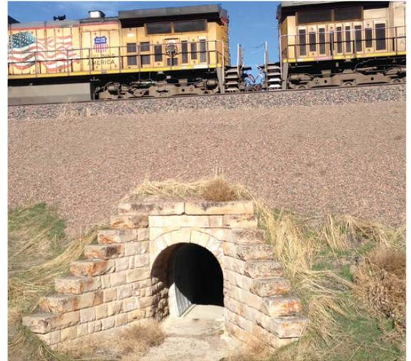
Contech Tunnel Liner Plate was used to fully restore this pedestrian underpass directly under a fully operational rail line.
