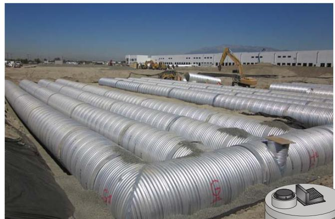
*CMP Detention Systems are customizable - may be designed for heavy loading and high maximum cover. Pretreating with a CDS hydrodynamic separator can increase longevity of the system.*
