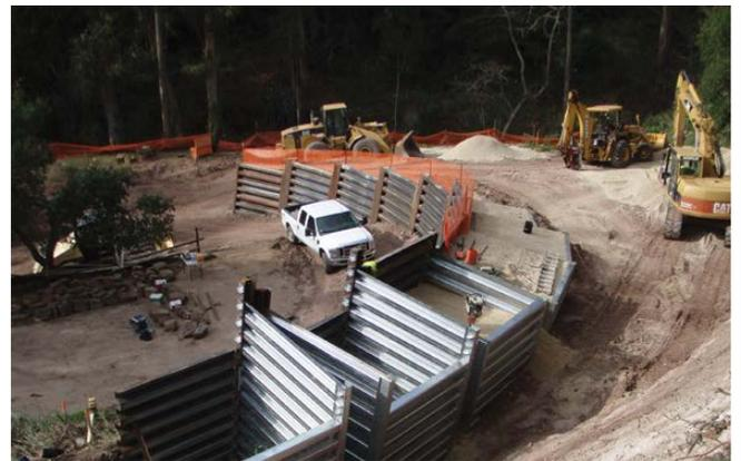
*Retaining Walls – Bin-Wall is a lightweight steel that is easily assembled to fully enclose fill material for a solid wall solution.*
