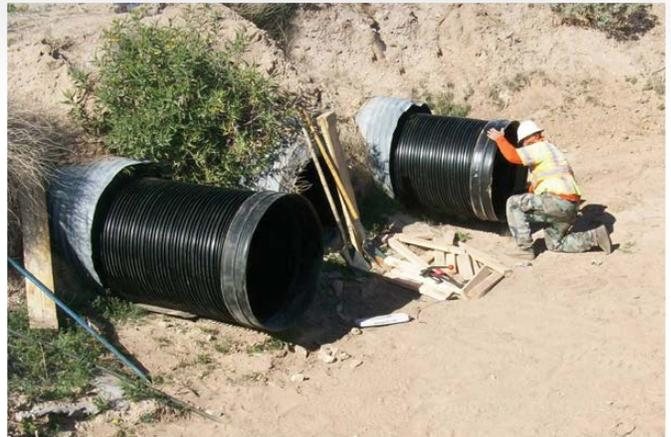
*DuroMaxx Steel Reinforced Polyethylene (SRPE) pipe is slip lined to provide a structural lining.*
