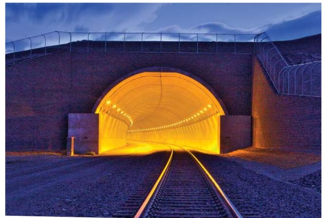
*Railway Tunnel – This BEBO structure allowed enough clearance to accommodate the construction of a second railroad track.*
