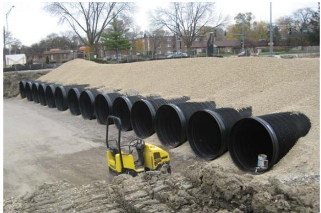
DuroMaxx Steel Reinforced Polyethylene (SRPE) pipe.
