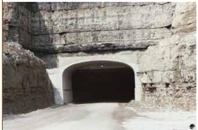
**Sugar Creek Mine (MO)** — protection from falling rocks (CON/SPAN)
