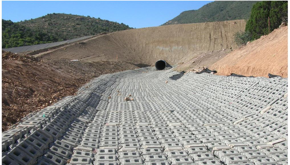
In the process of constructing the Carlota Copper Mine, Quadra needed to create a diversion channel for a large stream and eight other tributaries in the canyon. Originally, the channel was designed to be lined with shotcrete. After reconsideration of water velocities, differential settlement issues and long term maintenance, it was decided that articulating concrete blocks (ACB) would be the best solution.
