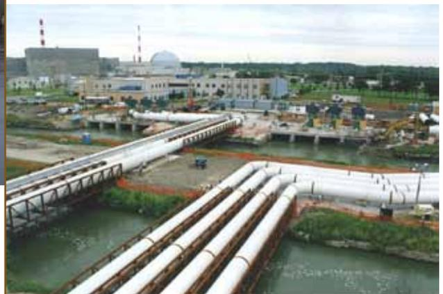
**Multiple Structures** — support 72" diameter pipes carrying extreme temperature liquids at a nuclear facility
