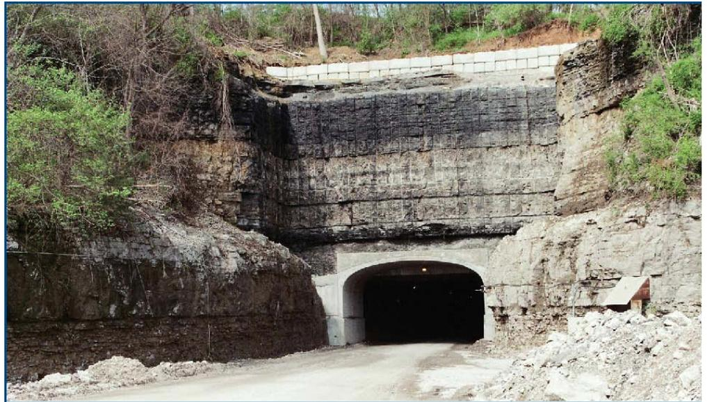
Due to the concerns of falling rock at one of their limestone facilities, LaFarge North America (LNA) needed to secure the mine entrance from debris as soon as possible.
