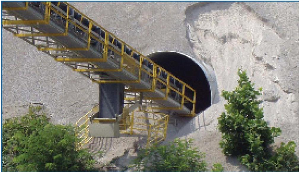
The Rogers Group needed a solution that could accommodate a conveyor system for a rock quarry in Louisville, Kentucky. Contech provided a 14' diameter MULTI-PLATE structure designed with external ring stiffeners/ring beams, and 96 feet of 48" corrugated metal pipe utilized for the escape tunnel. The height of the pile will not exceed 60'.
