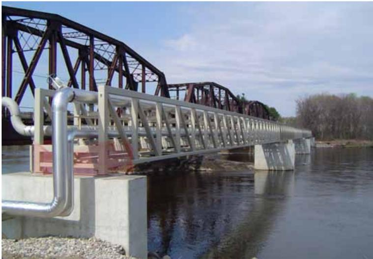
**Long Span Solutions** — single truss pieces can be combined to span large areas or waterways
