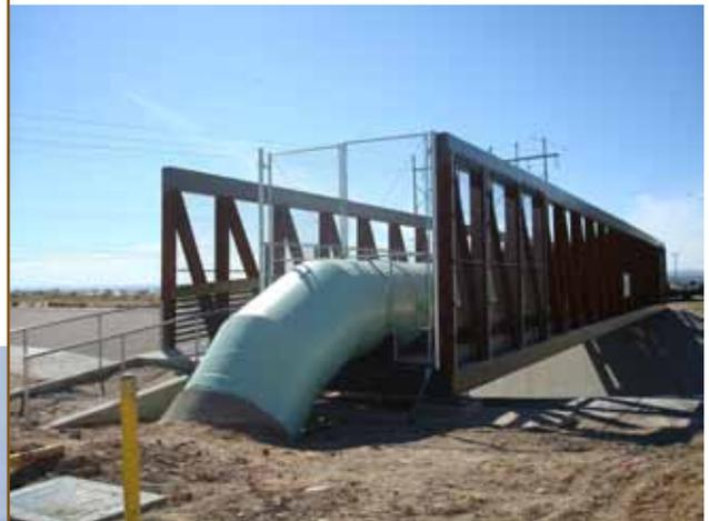
**Dual Applications** — pipe support structures may also provide necessary pedestrian walkways
